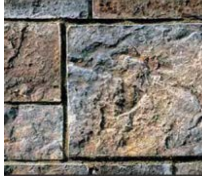
1 cm Derzli 1 cm Grout Joint
