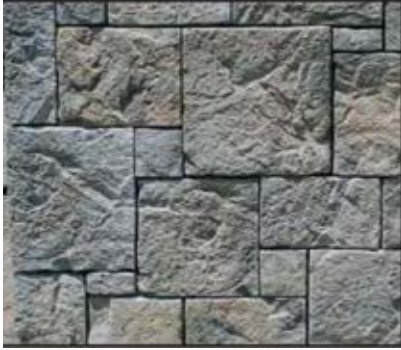
Kuru Yığma ( Derzsiz ) Dry Stacked ( No Grout Joint )
